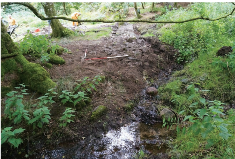
Photo 3. Water channel possibly cutting wall [A].
