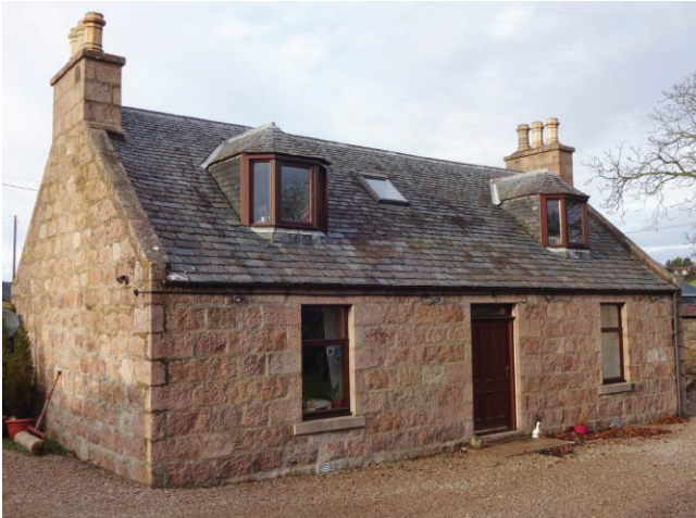
Photo 4. Broadsea. This is a much larger house than Burnside of Braco. Note the blocks on the front are all well-dressed, quarried stones whilst those on the gable end are field stones. (Photo by the author)
